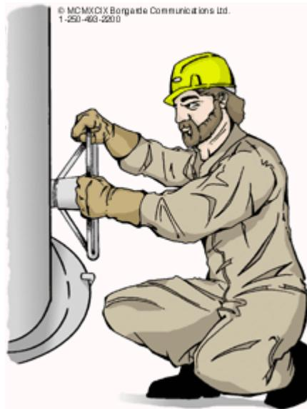
Fortunately, these hazards can be avoided through the use of lockout/tagout procedures. An employee performing the work places a lock and tag at any point where the equipment can be turned on during repairs or maintenance.
